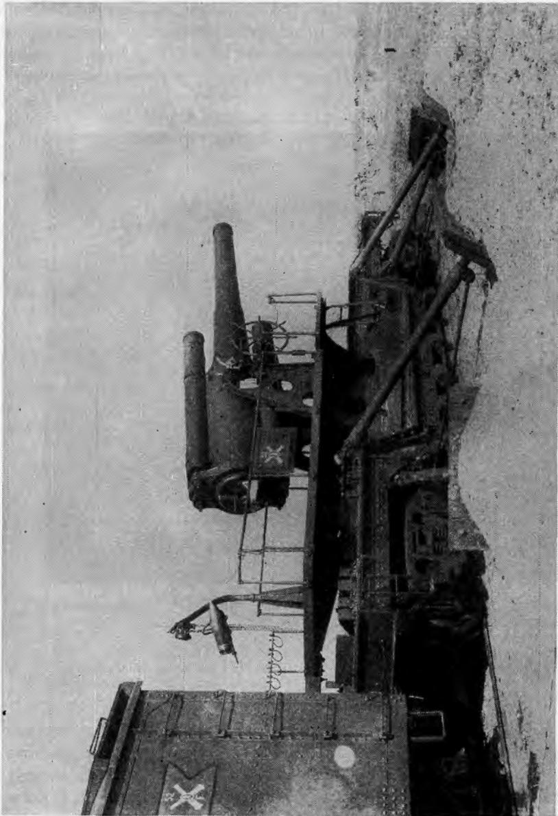
FIGURE 98.—8-inch gun on railway mount, M1918, emplaced.
