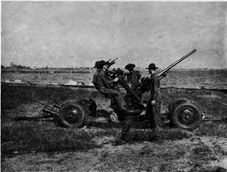
FIGURE 200.—37-mm automatic cannon on trailer mount in firing position.
